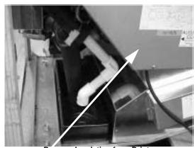
Remove Insulation from Driptray Drain Line Assembly
